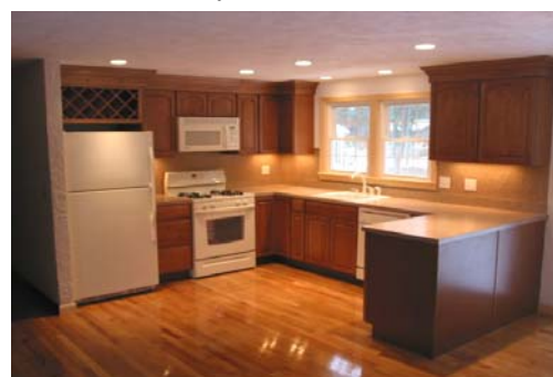
Full Kitchen Remodel & Hardwood Floors
