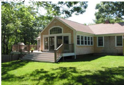
Sunroom Addition & Composite Deck
