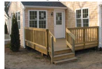
Pressure Treated Deck
